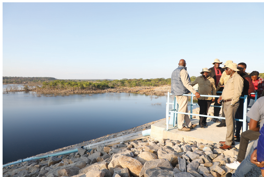
Chivhu Dam will improve food security in Mashonaland East through irrigation support
